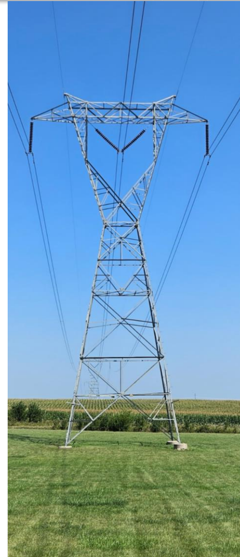
Existing 345 kV lattice structure
